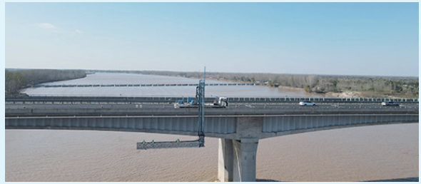
杭绍台桥梁定检
